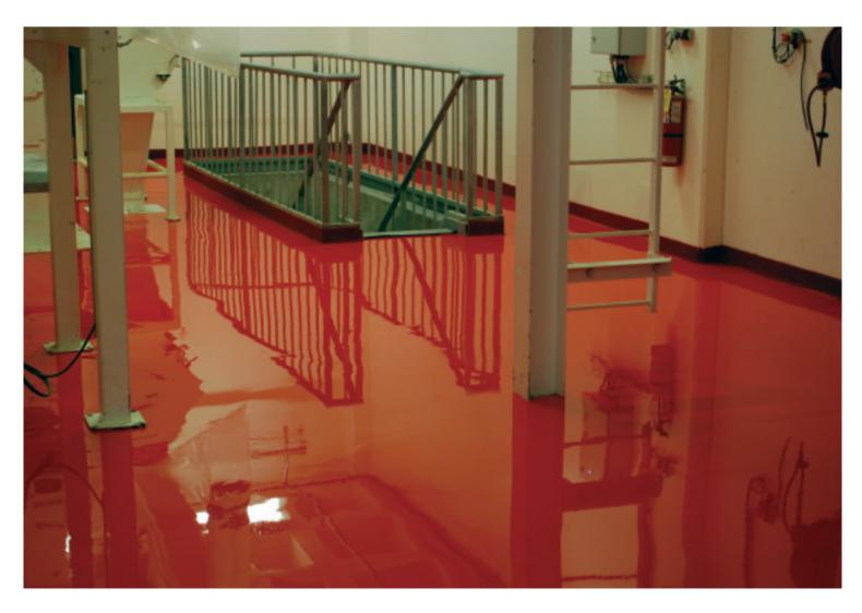
porosity of the concrete can generate harmful vapours in the building or can allow hazardous agents into the surrounding soil and ground water. AIF has been able to treat these slabs with a proprietary system that reduces porosity and restricts the movement of dangerous chemicals. The company recently completed 300,000 feet for a light bulb manufacturer in Oakville in order to reduce the risk of mercury contamination in surrounding areas.
